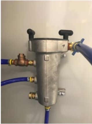
CHIP TRAP MANIFOLD
